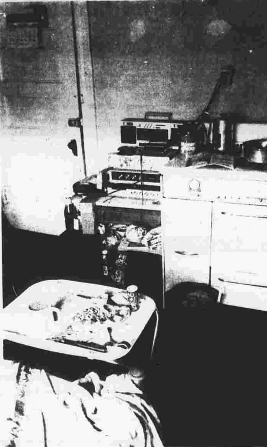
Bed, stove and stereo are squeezed into this one-room apartment at 801 Main St. A number of appliances are plugged into the electrical outlet above the stove. Under the town housing code, efficiency apartments are prohibited.
