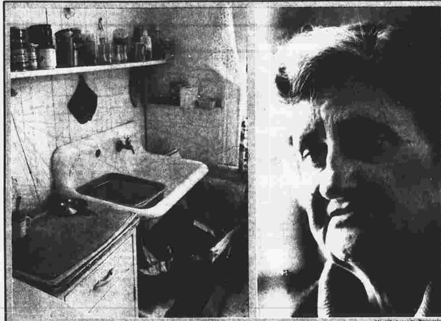
This cramped kitchen at 791 Main St. lacks hot running water, which is in violation of the housing code.
